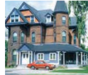
Former Lakeshore PPH, Cumberland House (Superintendent's residence), ca.1987, in adaptive re-use as a residence for a community health agency – the Jean Tweed Centre for women and their families with substance abuse and gambling problems.
